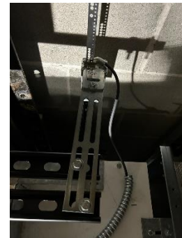
Figure 10: Sensor Mounting Plate Crosshead Installation
